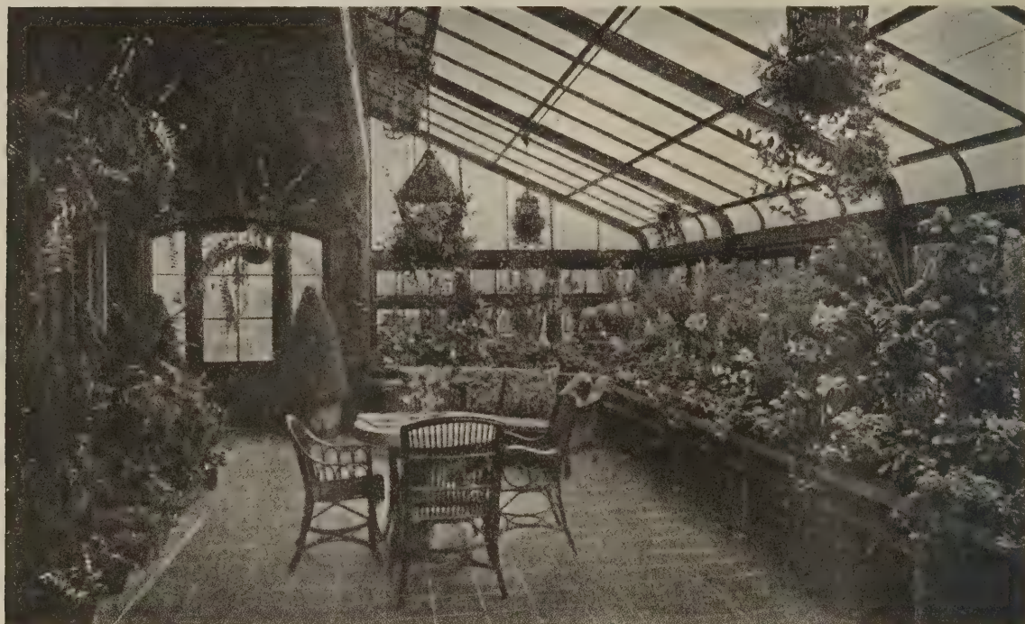
Interior of lean-to. Ample provision for sunlight is made. The tile floor simplifies the watering process. Note the steam pipes below the flower benches, much preferred to radiator heating
